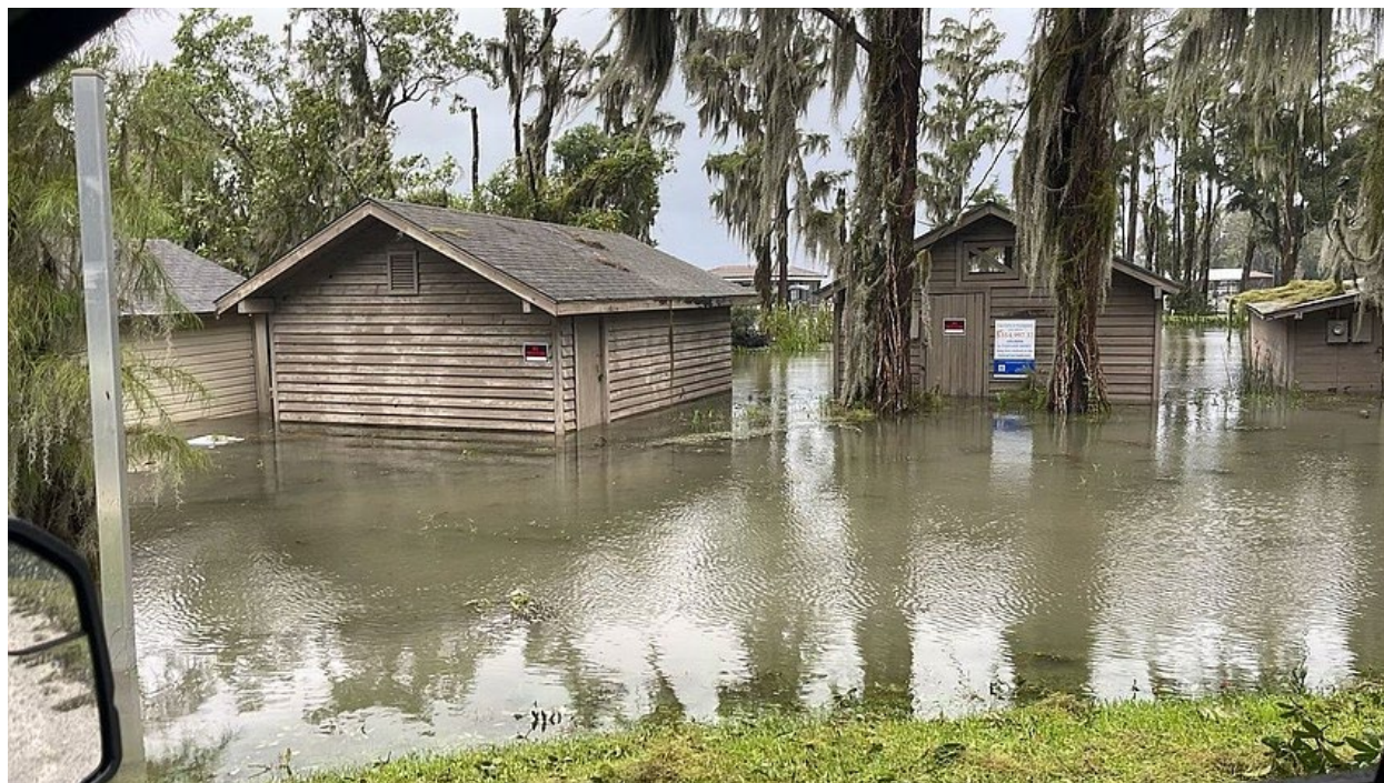
Figure 1. Flooded Boathouses in Windermere Partially Submerged After Milton. Photo credit: West Orange Times Observer.
