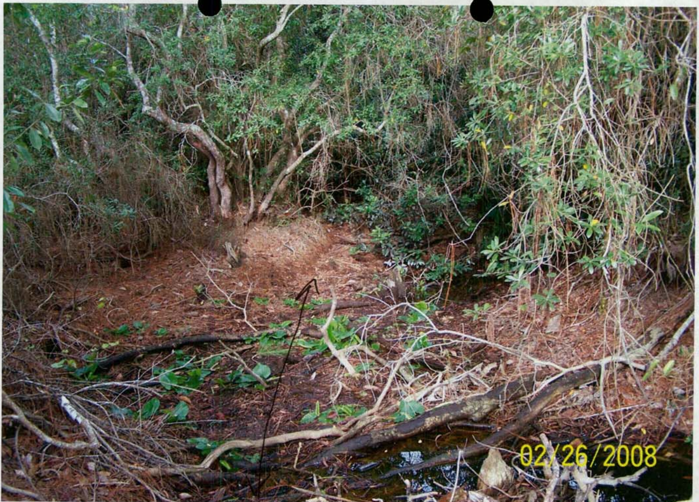
Ditch connection facing west
