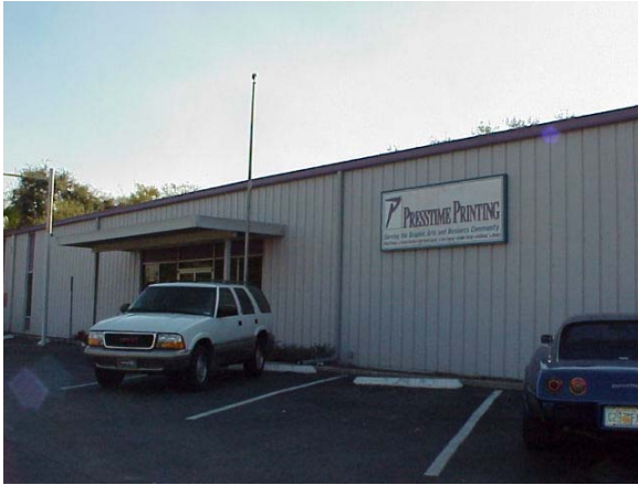
Example of prohibited material Corrugated metals as a primary exterior building material are prohibited.
