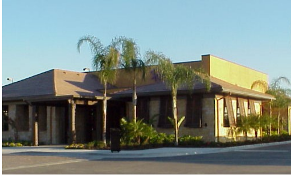
Example of primary façade for commercial use This primary façade is attractively landscaped with clusters of palms. It eases the transition from the horizontal surface of the parking area to the vertical height of the structure.
