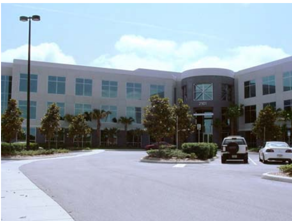
Example of a highly-visible customer entrance with accompanying landscape.
