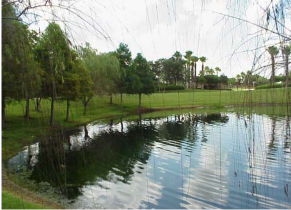
Example of a stormwater pond as a visual amenity
