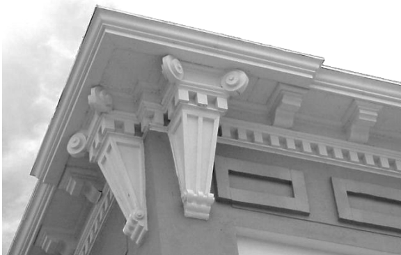
Example of cornice and ornamental detail
